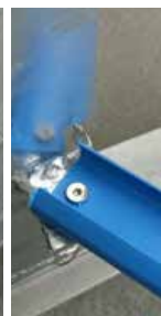
Installation of floor rail connector
