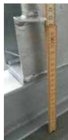
Installation depth of steel girder (approx. 22.5 cm)
